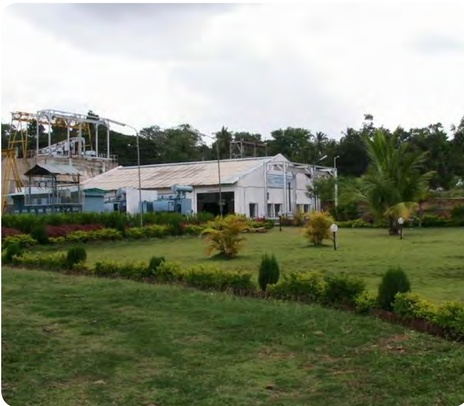
The Akkihebbal project harnesses hydropower to generate clean electricity
